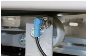
Handrail speed detect
