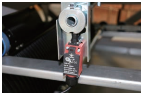
Step collapse detect
