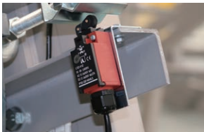
Step chain loosen and broken protection
